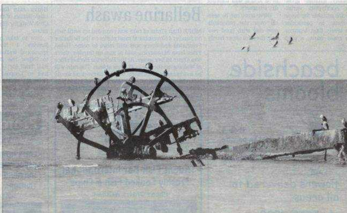
Paddlewheel: All that remains today of the great paddle steamer Ozone at Indented Head, 82 years after the hulk was sunk just offshore to form a breakwater. —PHOTO BY GREG WANE
