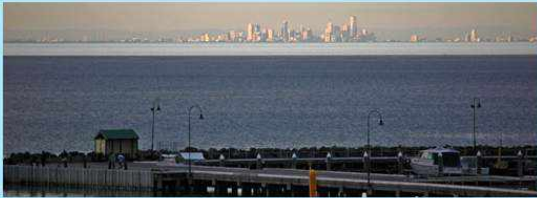
BELLARINE FERRY AND PORTARLINGTON SAFE HARBOUR
